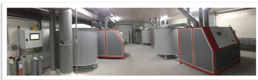
3 x ST1000 + VSA Type 60 + CMS system for 30 x 200 CA rooms for pears.
